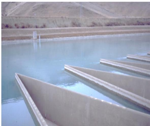
**Figure 1:** Triangular labyrinth weir of hydraulic power plant of Ohau C in New Zealand
