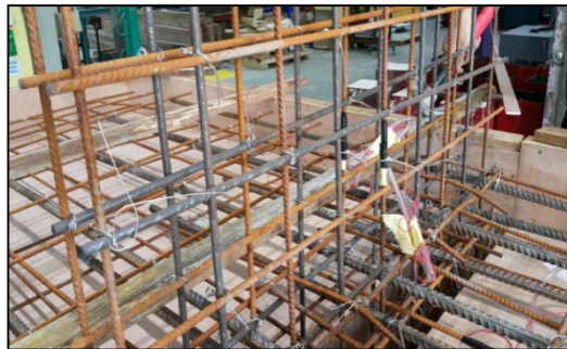
Figure 3: Reinforcement detail of Interior Wall-slab joint
