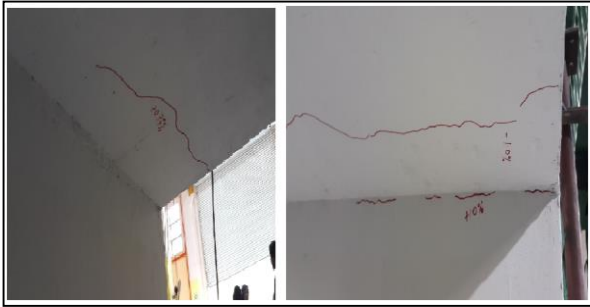
(c) Slab panel surface
